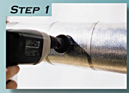
**CUT HOLE WITH HOLE SAW**
